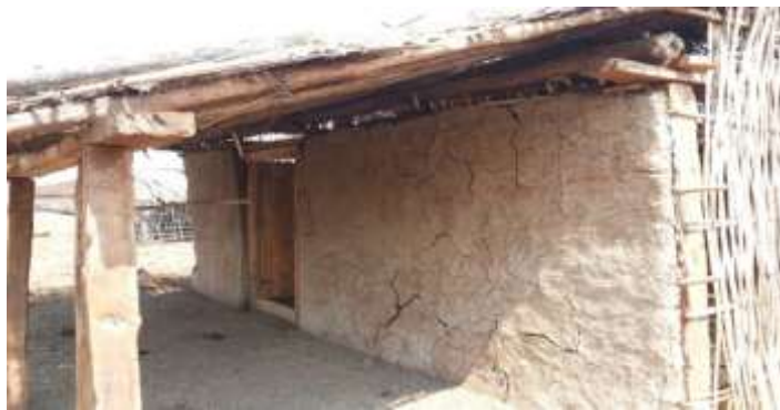
View of traditional hut in Rajaborari village
