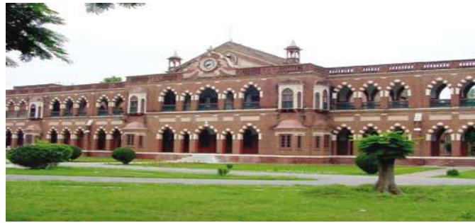
Figure 3: View of REI Building, oldest educational building in Dayalbagh
